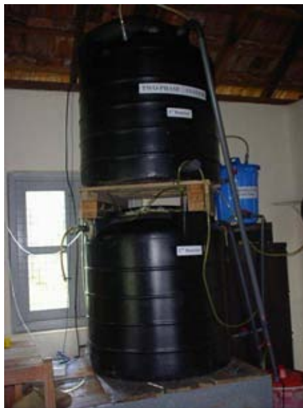
Fig. 4: Designed and fabricated two-phase reactor system
