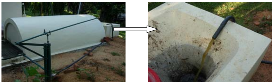
Fig. 6: Appearance of the 3B type bio gas plant
