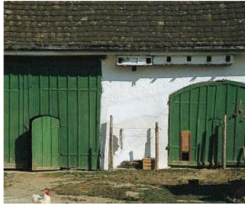
On unsealed courtyards precipitation can percolate naturally.
