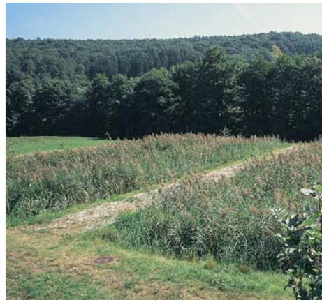
In small settlements it makes sense to establish simple and decentralised waste water treatment plants. In the root area of this waste water treatment wetland the effluent is filtered.
