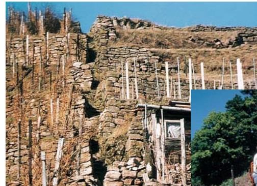
Redevelopment measures in the vineyard: The new wall has also been constructed as a dry-stone wall. It provides cover for numerous thermophilic species.
