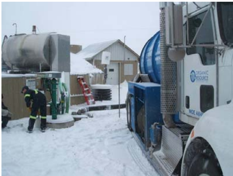
Fig. 2: DAF being unloaded into holding tank. Stainless steel tank heats DAF to 70 degrees C for 1 hour
