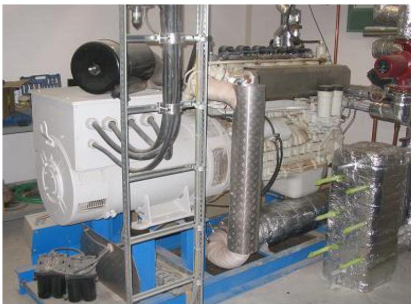
Abb. 2: Foto BHKW 1 (Gas-Otto-Motor, 190 kW el. )
