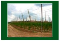
The wirework was not fully loaded by vigorous hop plants in the first vegetation year. Nevertheless, deformation of soil under poles was obvious. Therefore the wirework had to be fastened after harvest. In 2007 measurements of forces in anchor connecting rods were repeated.
